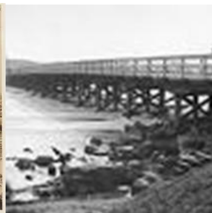
1861 Yarra Falls Bridge near Queens St
